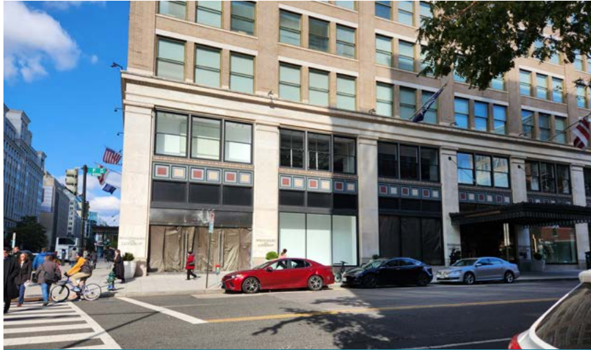
F STREET ENTRANCE
