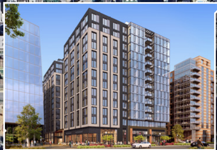
1150 FIRST STREET NE
