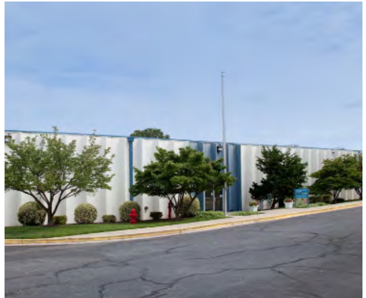
72,000 SF Manufacturing Building (Building A)
