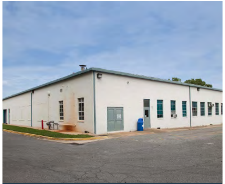
30,000 SF Warehouse (Building B)
